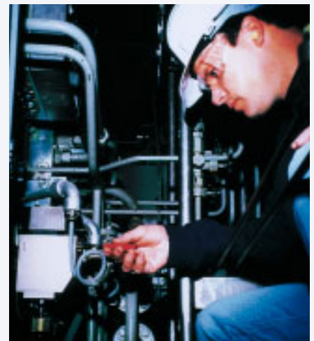
Minimum and maximum output pressures can be easily set externally.
